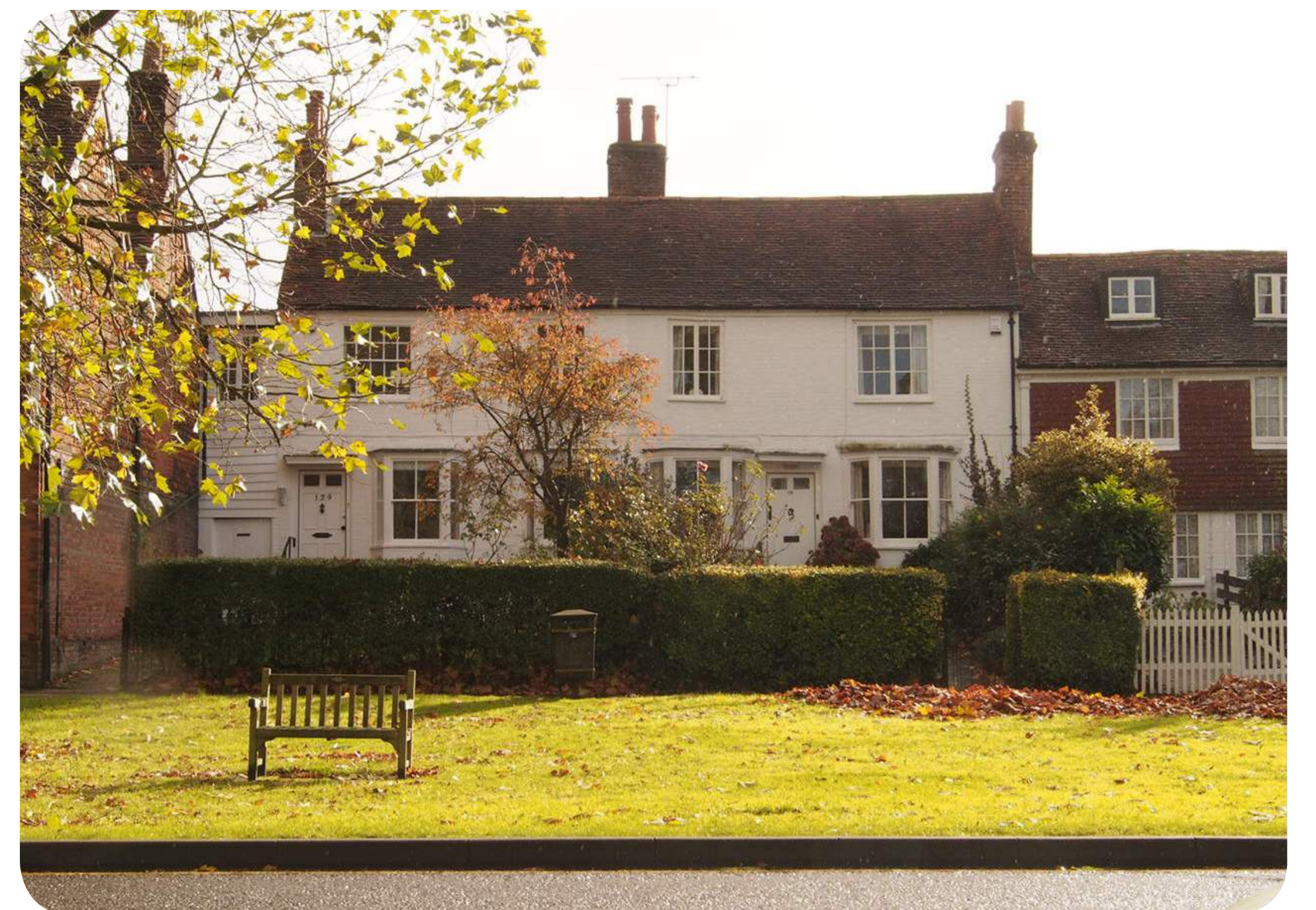
Tenterden vernacular architecture in the High Street
