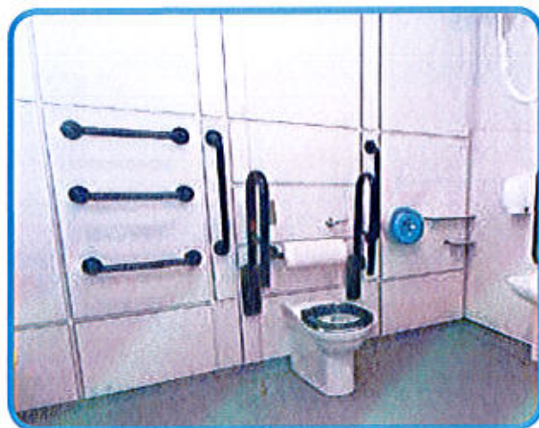
Peninsular layout WC with transfer space and drop-down grabrails on both sides. Alarm cords should not be tied up and the transfer space kept clear
