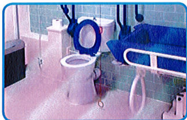
Alarm cord with bangles at two heights, which can be reached easily if a CP user or assistant has fallen onto the floor. The reset button should be easy to find and operate if the alarm is accidentally triggered
