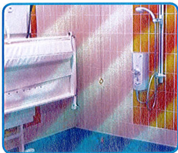
It is good practice to install an alarm in the shower area. The red cord and bangles should contrast against the background and should be easy to identify
