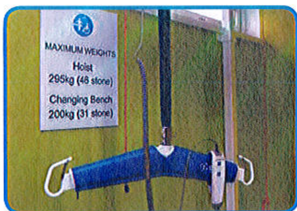
The East Midlands Airport have installed a hoist with maximum safe lifting weight of 295kg (46 stone) and included clear signage indicating capacities of the equipment
