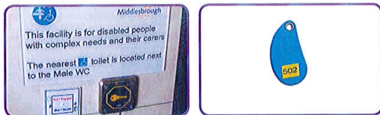
The fob reader (left) and fob (right) at Middlesbrough Bus Station's CP facility are designed to manage access while remaining user friendly
