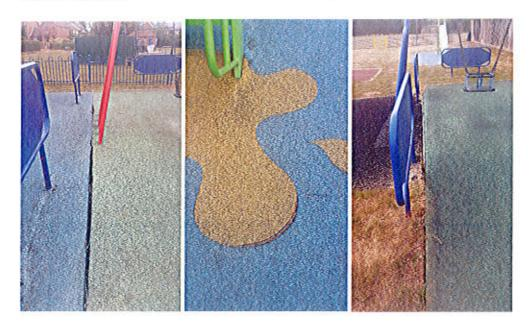
Although this is not considered to be dangerous it will continue to deteriorate over time. 'Vitaplay' have been to look at the surface and have provided a quote for repair. This is guaranteed for 12 months. A complete resurfacing would be guaranteed for 5 years but would be a considerable expense.
