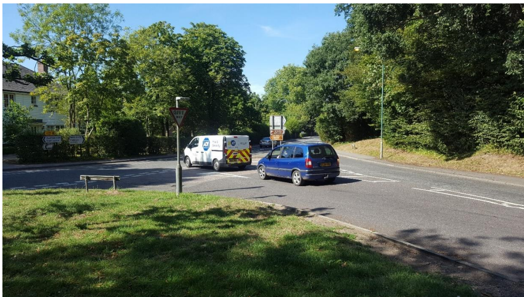
Figure 1: General view of junction from SE corner of Beacon Oak Road and Ashford Road
