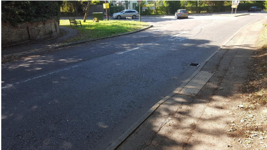
Figure 3: View of uncontrolled pedestrian crossing in Beacon Oak Road
