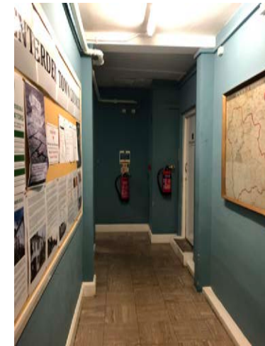
existing office corridor
