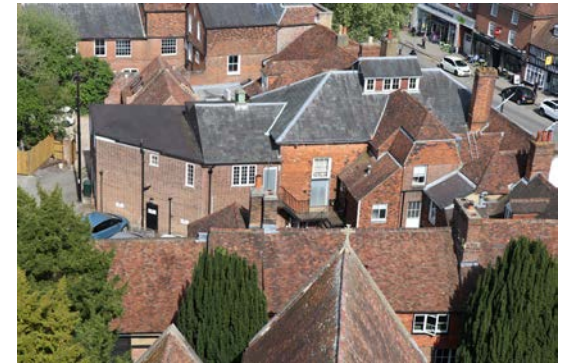
existing view from St Mildred's Church
