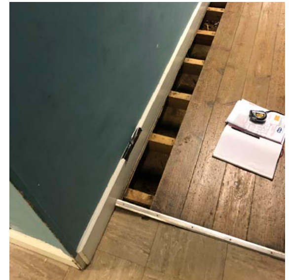
floor board removed showing floor construction
